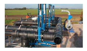
At Gemidan's pre-treatment plants, food waste is converted into a pure bio pulp. Their technology ensures a sustainable use of the waste, and AVK knife gate valves control the flow.
