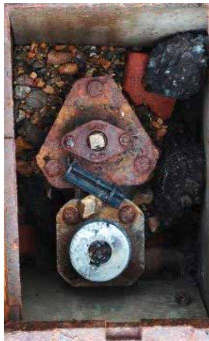
Existing hydrant with outlet security device installed
