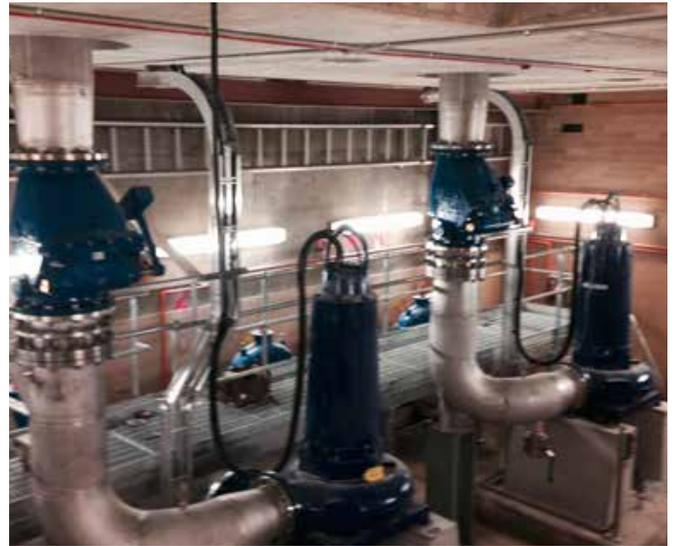
AVK Australia recently completed the valve supply of a major upgrade and refurbishment to the SA Water River Road wastewater pump station in Port Noarlunga. The valves included the series 55 RSGV, series 41 RSCV, actuation and other ancillary valves.
