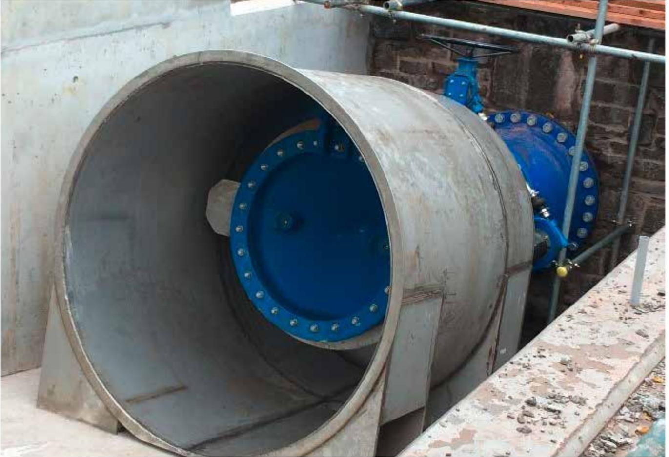
Picture 1: Free discharge valve and hood installation
