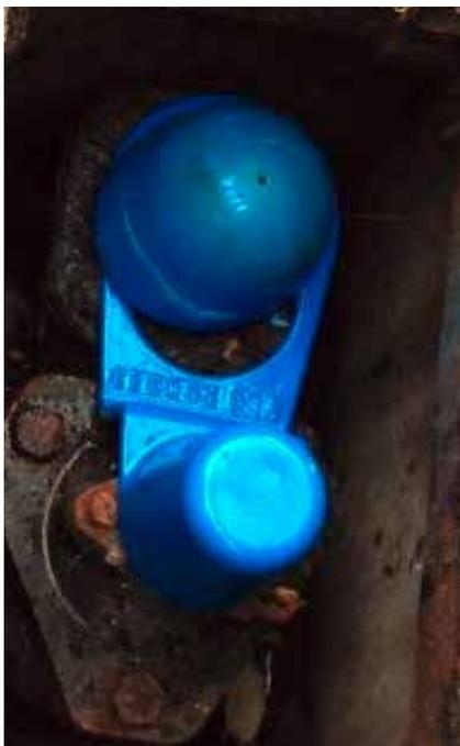
Existing hydrant with AVK device fully installed. Note the outlet and operating cap now fully protected
